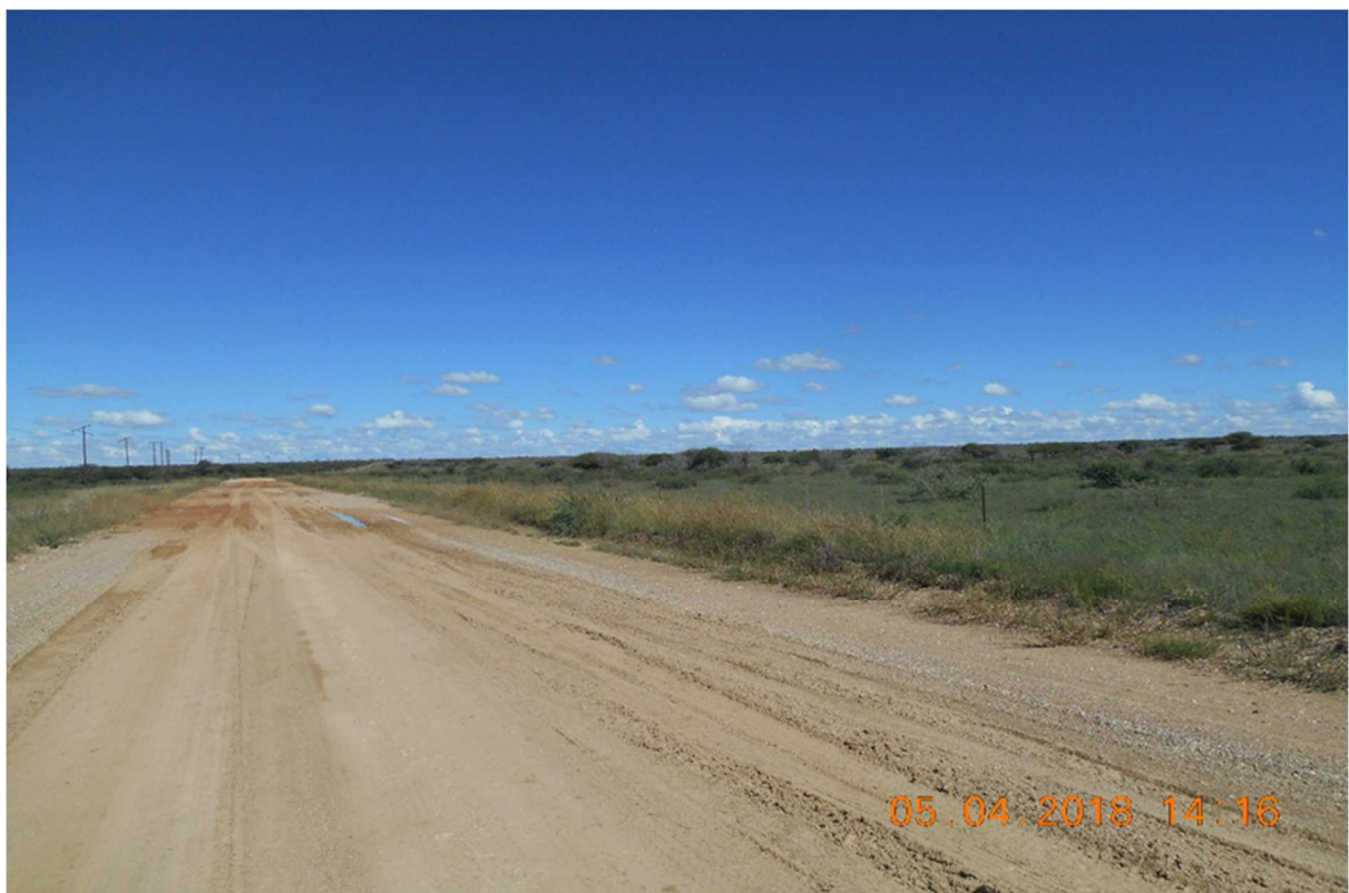
Figure 25: Gravel Road in the Vicinity of Stella
