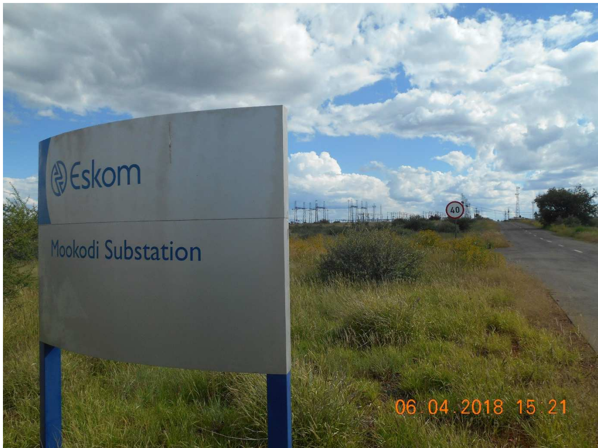
Figure 29: Existing Mookodi Substation
