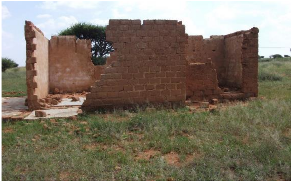
Figure 10: Remains of brick structure
