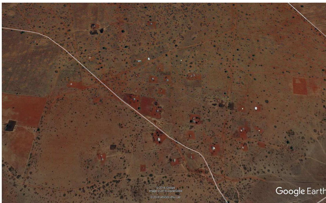
Figure 11: Impacted Structures in Lokgalong [S 25 44 40, E 25 30 48]
